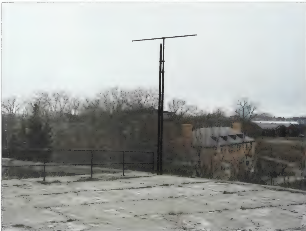
Figure 3.31. View looking northwest at metal pole, Battery Potter. A T-shaped metal pole is located north of the fire control stations and was used in observing and recording weather phenomenon (Olmsted Center, April 2008).
